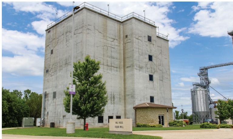
Hal Ross Flour Mill – state-of-the-art pilot scale flour mill used for teaching, research, and industry training on full-scale equipment and control systems found in commercial flour mills
