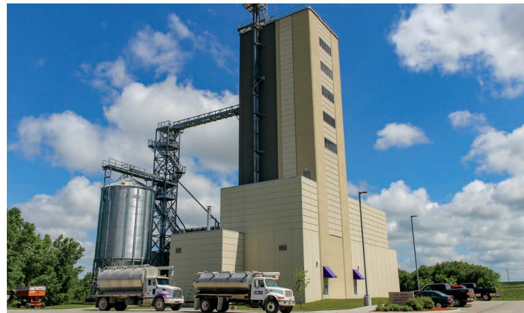
O.H. Kruse Feed Technology Innovation Center – a modern feed mill used for teaching feed production, pet food development, grain handling, and featuring an embedded BSL-2 research facility
